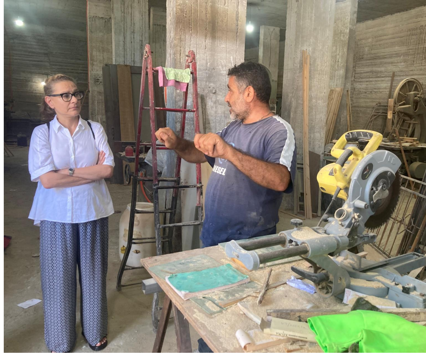
MECC rehabilitation Project in Sidon
